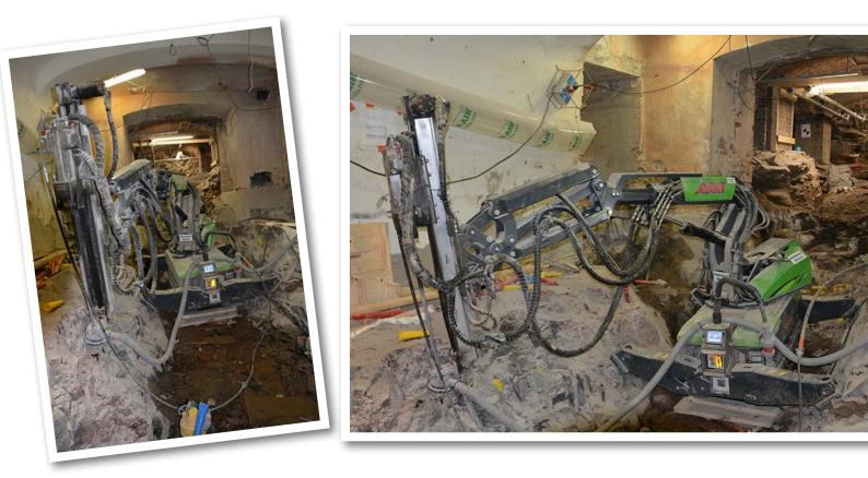
he renovation started last November and will last for a total of two years. In addition to a thorough interior conservation, the first floor is expanded for extra rooms as well as space for heating, ventilation, air conditioning and other building service equipment. The first floor stands on top of granite bedrock, which requires 500 m<sup>3</sup> of rock to be removed.
